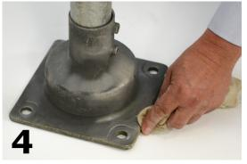
• Adhesive will come out the sides. Use a rag to wipe excess. Wait 24 hours for adhesive to be fully cured
